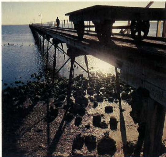
Jetty at Ceduna, the last main township on the road west across the Nullarbor Plain.
